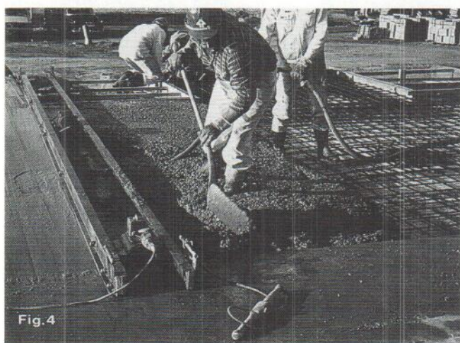
Fig. 4. Concrete workers laying a floor.
