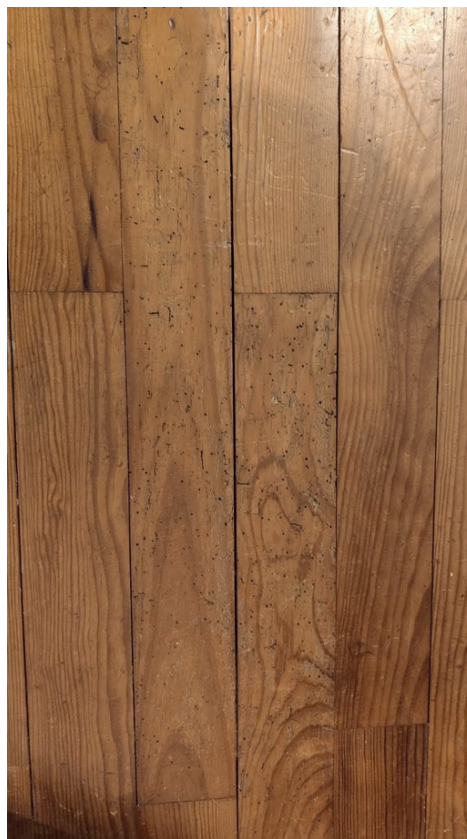
Fig. 2. Photograph showing indirect proof (holes) of the presence of the wood-boring beetle ( Anobium punctatum ) in the old wooden floor of the child's bedroom.
